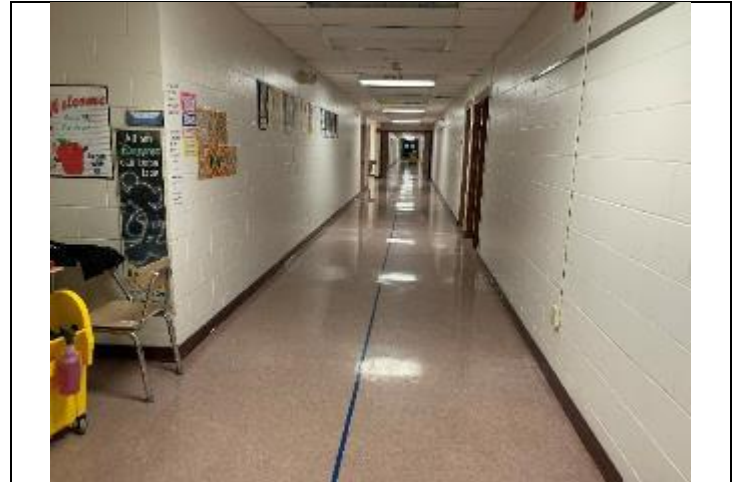
8. Hallway with CMU walls, 12" tile and suspended ceiling tile.
