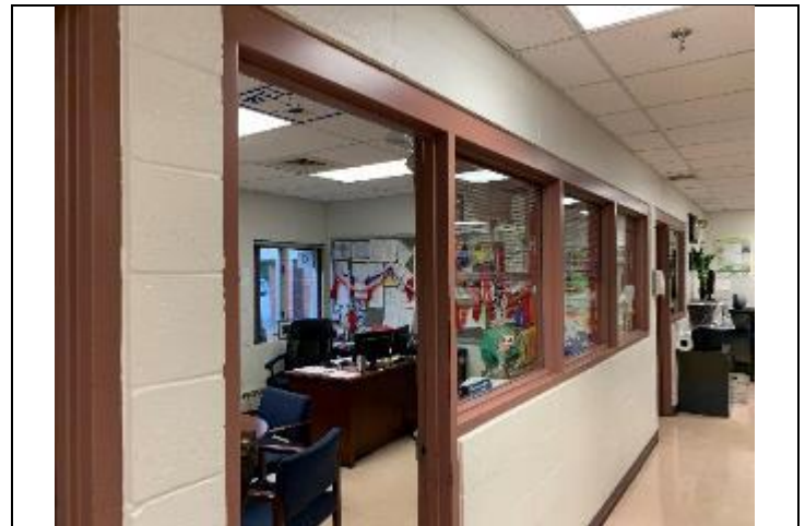
6. Main office with CMU walls, 12" floor tile and suspended ceiling tiles.
