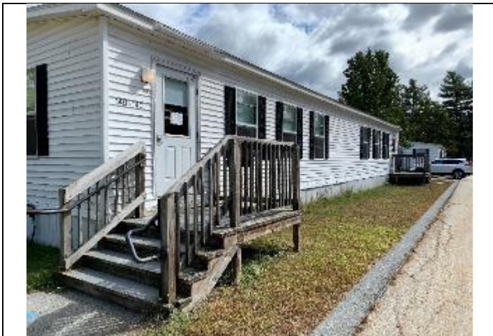
5. Detached modular classroom structures.
