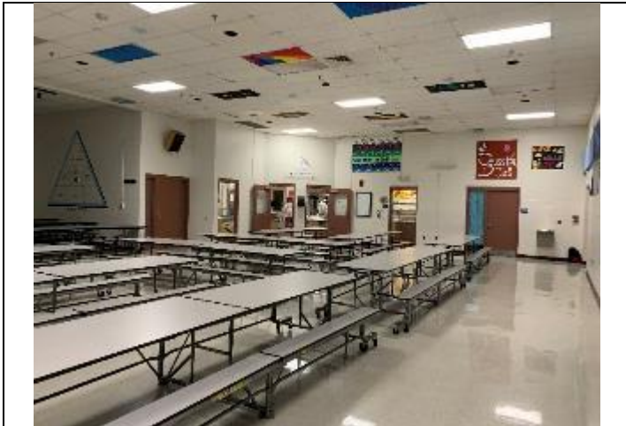
11. Cafeteria with 12" tile and suspended ceiling tiles.
