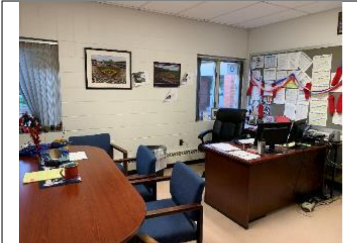
7. Main office with CMU walls, 12" floor tile and suspended ceiling tiles.
