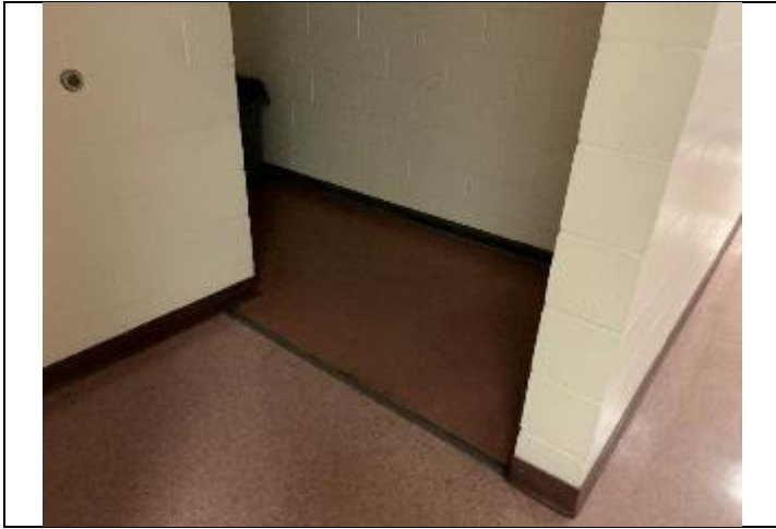
13. Poured flooring within hallway bathrooms.
