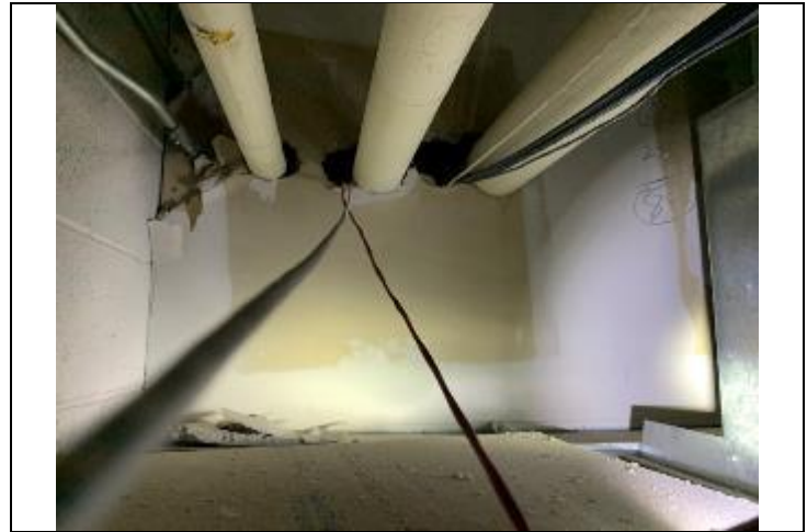
18. Gypsum and Joint compound present above hallway ceilings.
