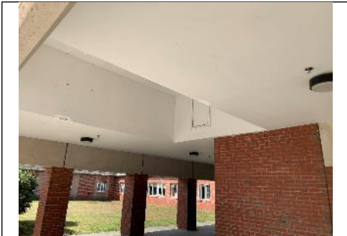
3. Entry overhang with gypsum and joint compound.
