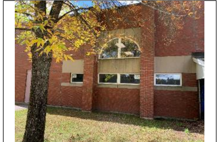
2. Exterior Windows with white caulking.
