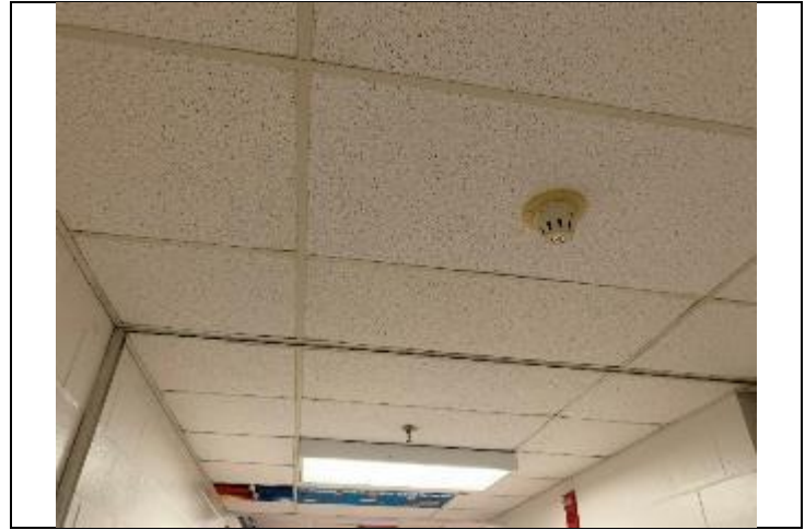
14. Suspended ceiling tile was present throughout with LED lighting.
