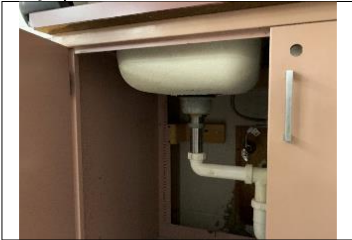
17. Sink Basin undercoat. No asbestos detected.
